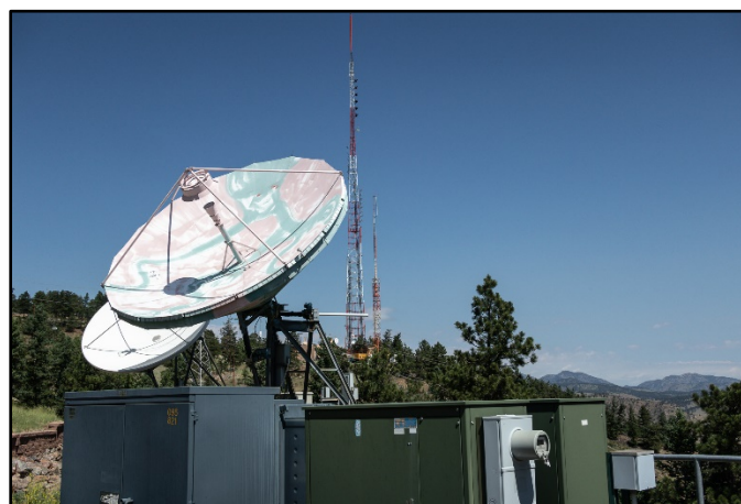
Figure 5 Lookout Mountain Communication Towers
